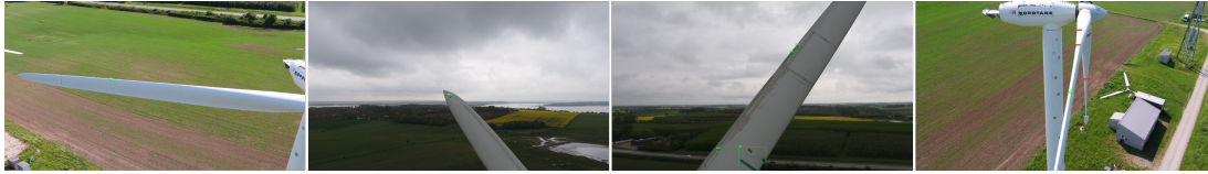
Figure 3.4: The figure shows model outputs for four images from the DTU dataset. The three images on the left demonstrate successful anomaly detection and localisation, while the image on the right illustrates failure cases when anomalies are at the edge of the object.
