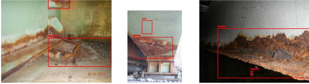
Figure 1.2: Supervised anomaly detection models can misinterpret defect types when context and material properties are not considered. In this example, the model mistakes corrosion for concrete spalling
