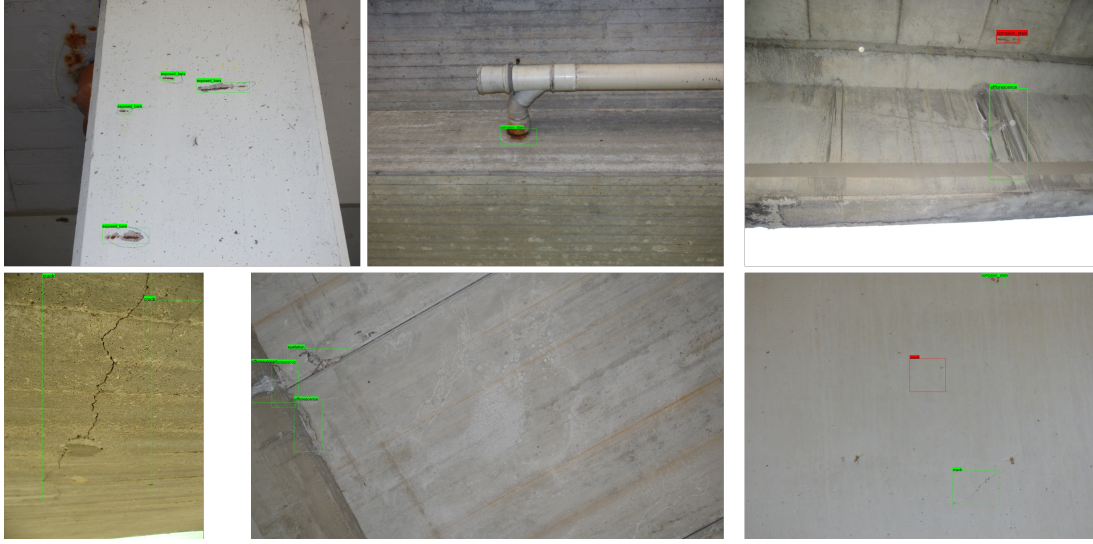
Figure 3.3: Anomaly detection results on CODEBRIM dataset. The figure shows model outputs for six images. The four images on the left demonstrate successful anomaly detection and localisation, while the two images on the right illustrate failure cases where not all anomalies are detected.
